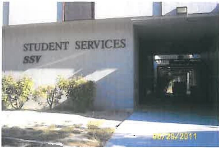
SSV Leading to Court Yard
